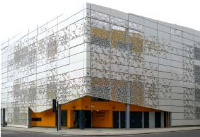
The new Rose Lane car park is only half full at peak times, although this may change if new office development materialises
