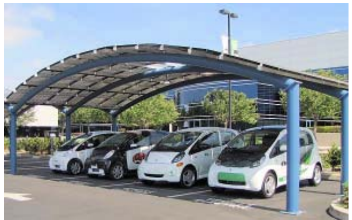
Research suggests that providing canopies carrying solar panels for the charging points can be advantageous
